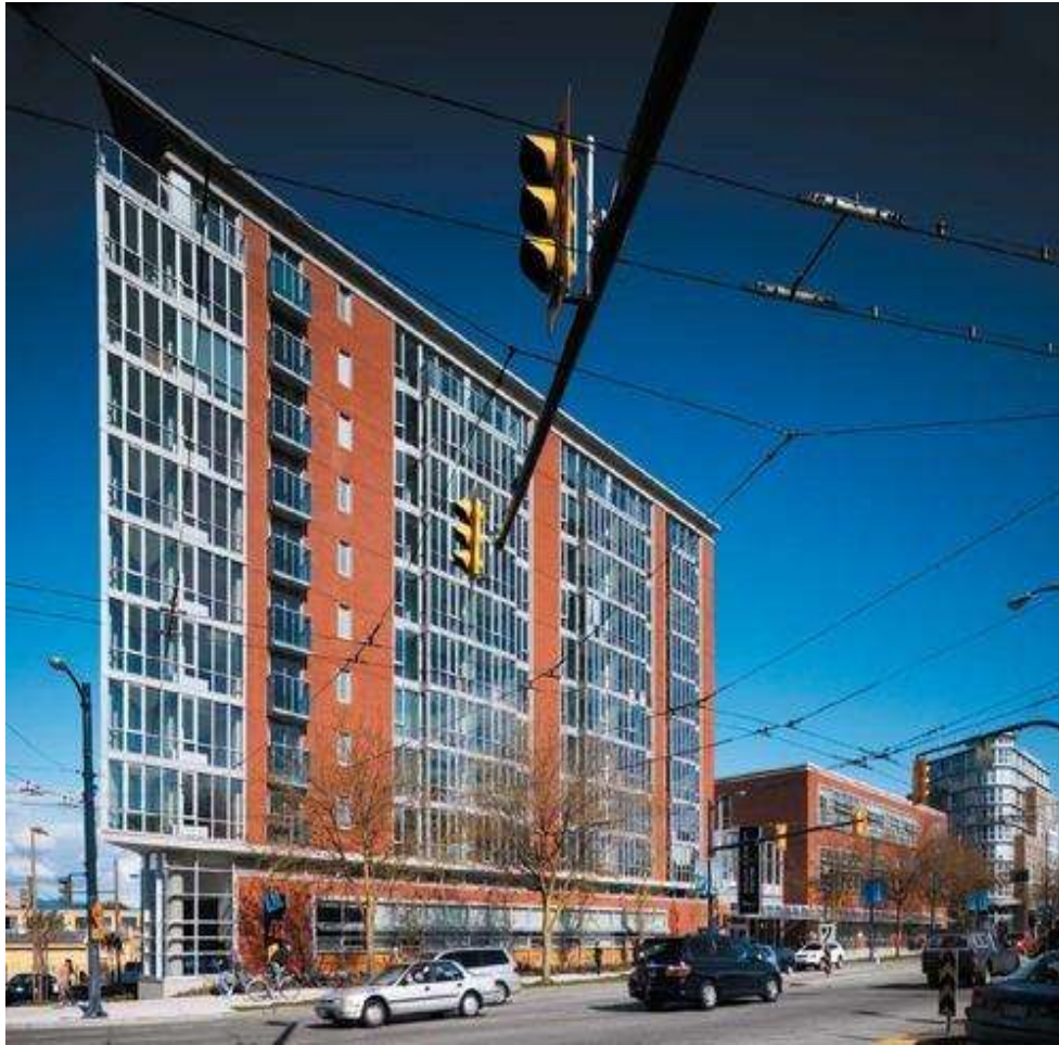
Figure 4. The Mount Pleasant Centre from Kingsway. The residential tower is to the left and the three-floors of community center to the right. © Martin Tessler
