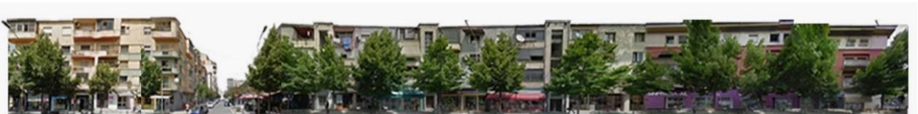
Figure 55. Third segment of elevations of the selected buildings (by author)
