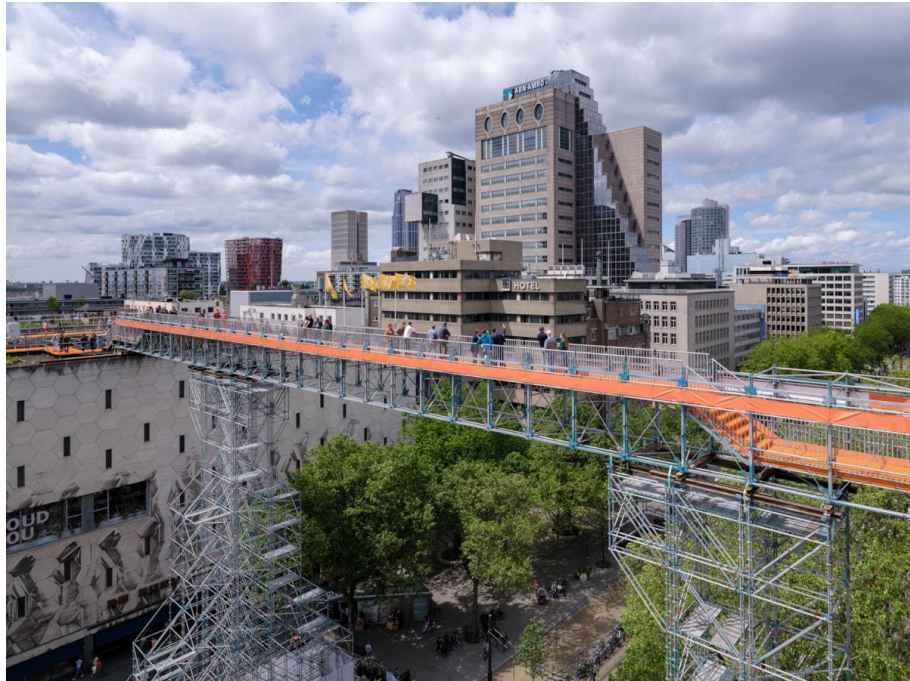
Figure 30. Rooftop Walk, picture taken from Dezeen
