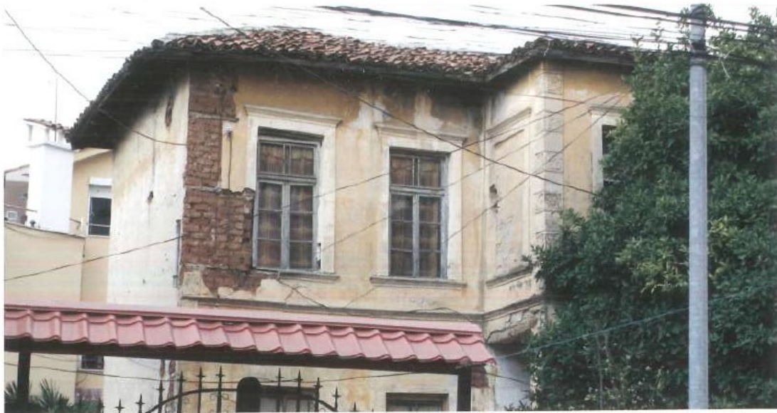
Figure 28: Adobe with linear beams
