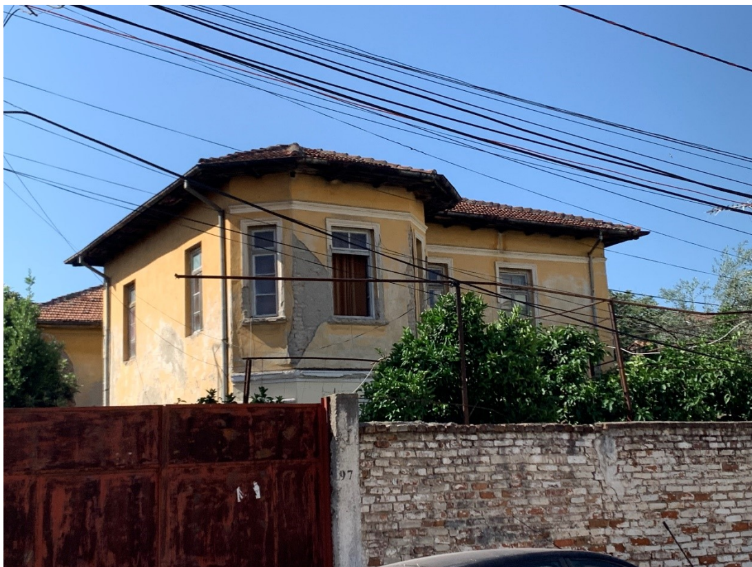
Figure 66: Villa nr.22 current situation (Source: Author, 2022)
