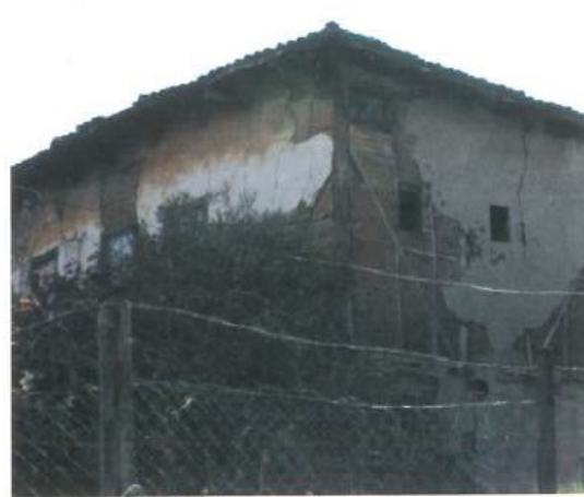
Figure 30: Adobe with crossed beams
