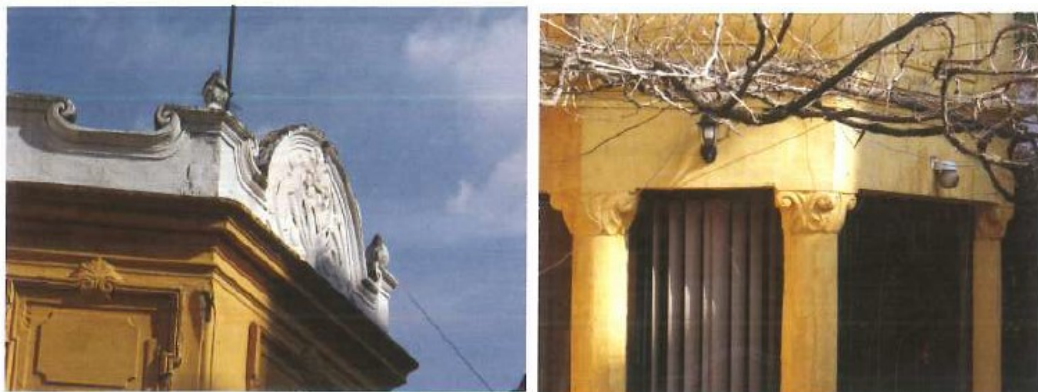
Figure 56: Architectural details applied on Villa nr.13 (Source: Vilat e Tiranës, Dr. Vera Bushati)
