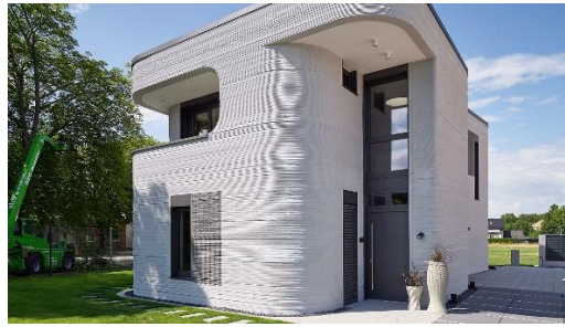
Figure 38. 3D printed house in Germany, image source [55]
