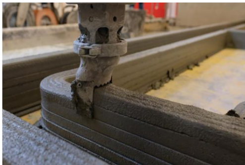
Figure 9. BOD2 3D Printer nozzle, image source [22]
