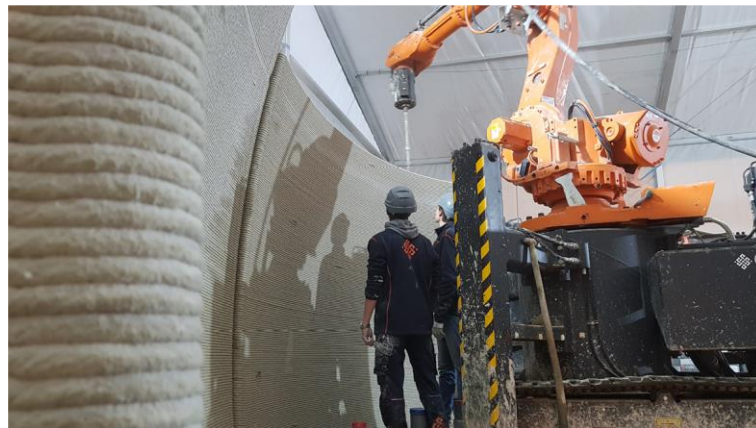
Figure 18. CyBe RC 3Dp, image source [32]
