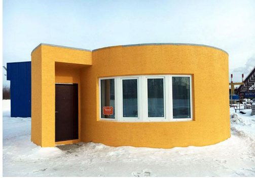
Figure 59. Apis Cor 1st 3D printed house, image source [77]
