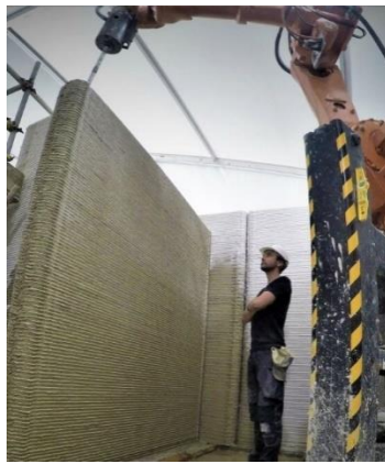
Figure 58. Saudi Arabia House walls, image source [76]
