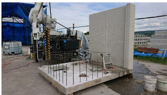
Figure 54. Toilet units steel bars, image source [73]
