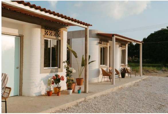
Figure 29. Two house units already finished, image source [46]
