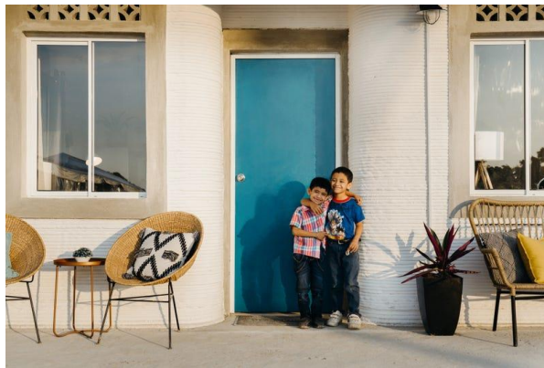
Figure 30. 3D-Printed walls, image source [46]
