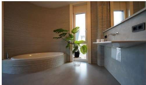
Figure 39. 3D printed house in Germany interior, image source [54]
