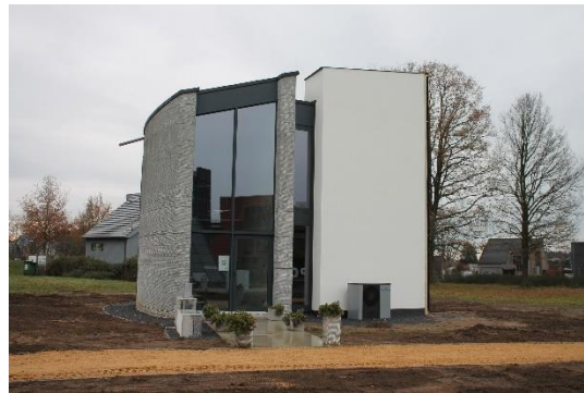
Figure 34. Westerlo 3D printed 2-storey high house, image source [50]
