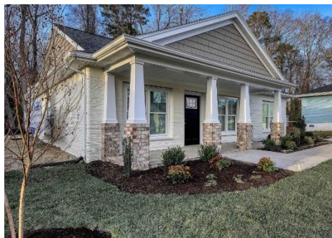
Figure 40. 3D printed house in Virginia, image source [57]
