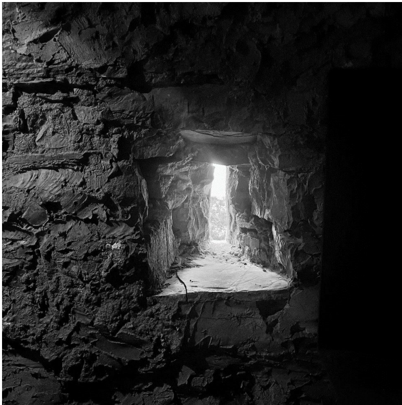
Figure 33: Opening in the wall to allow ventilation in “ahri” photo [24].
