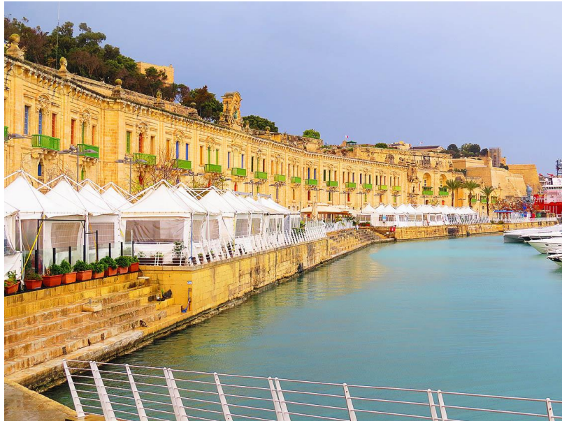
Figure 2. Valleta Waterfront general view (Source: Chevron)
