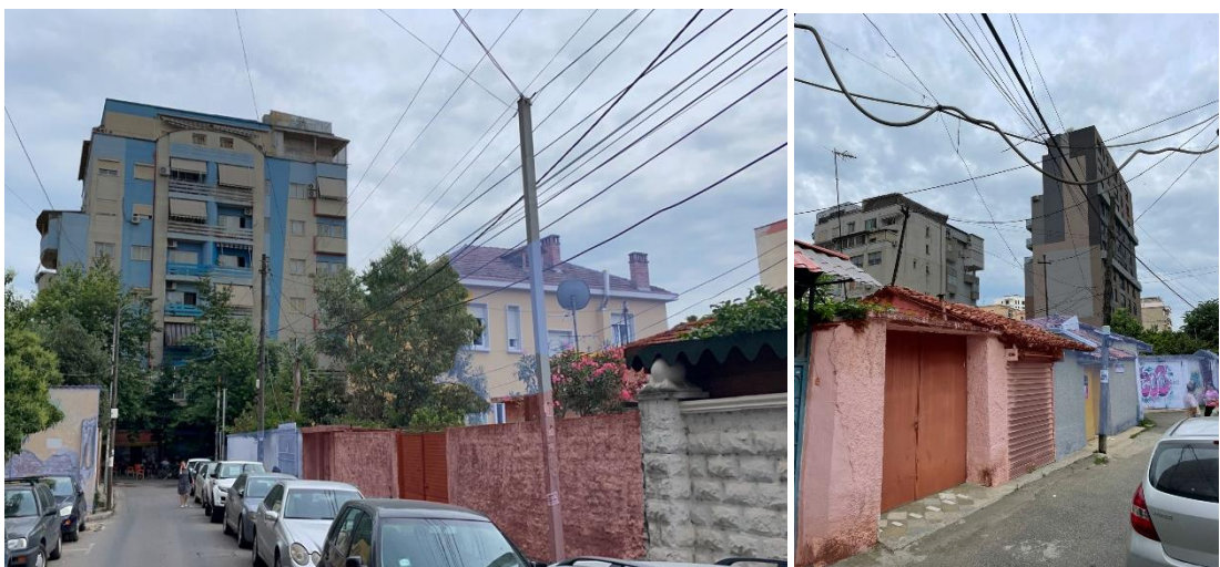
Figure 32. Left: Photo from Location 5, Right: Photo from Location 4: Pre-socialist ( red ), socialist ( blue ) and post-socialist ( black ) buildings (© Artea Zera).
