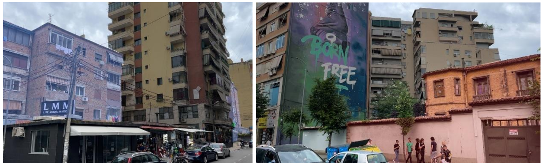
Figure 31. Photos from Location 3, Pre-socialist ( red ), socialist ( blue ) and post-socialist ( black ) buildings (© Artea Zera).
