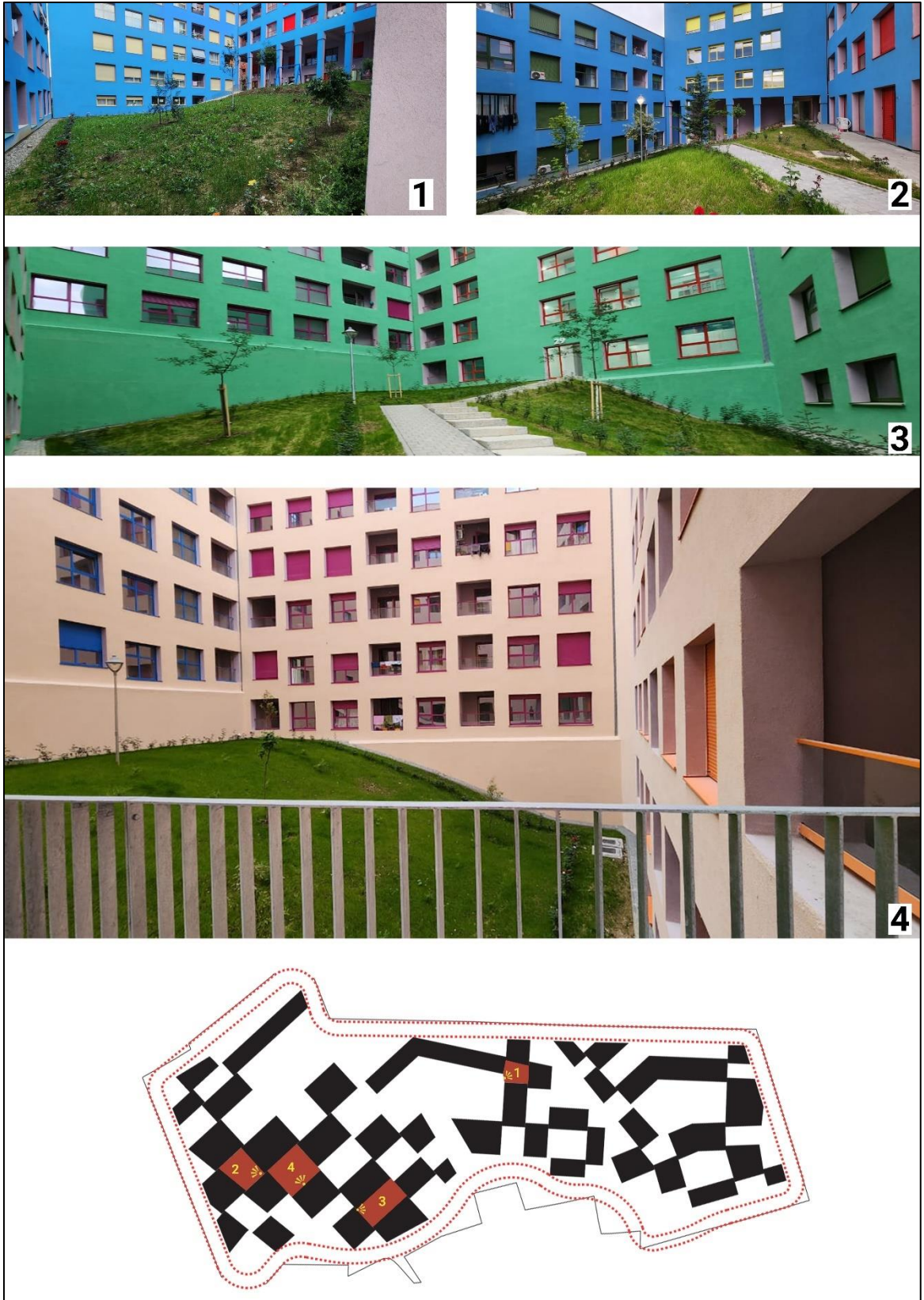
Figure 13. Photos taken from the closed courtyard part of complex (Author)
