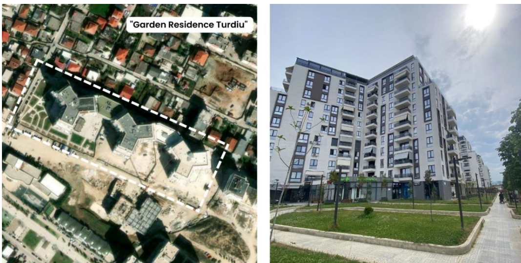
Figure 15. "Garden Residence Turdiu" Site
