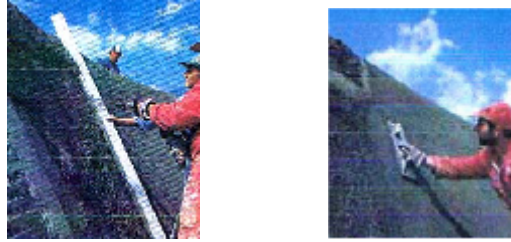
Fig.6. The cast in place and final smoothing the layer on the slope surface
