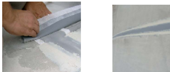
Fig.8: a/placing the PVC materials to protect the joints; b/the view of protected joints
