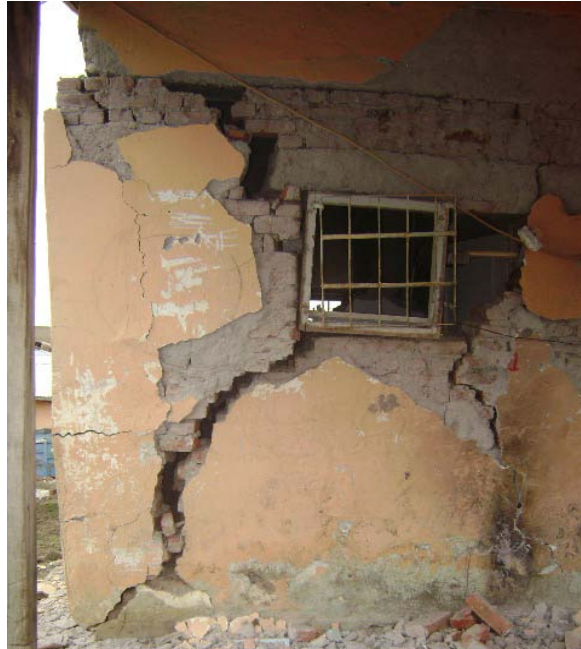
Figure 8 Wall opening close to the building corner
