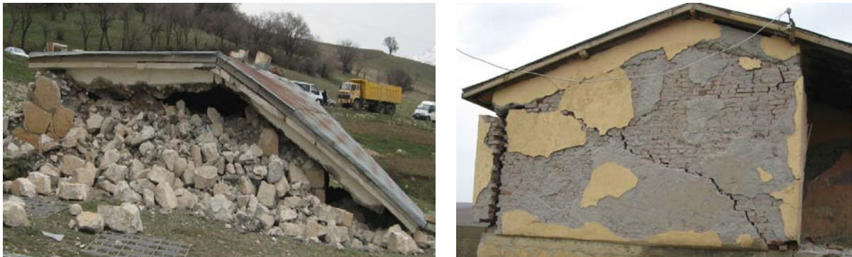
Figure 3 Heavy -saddle shaped roofing systems
