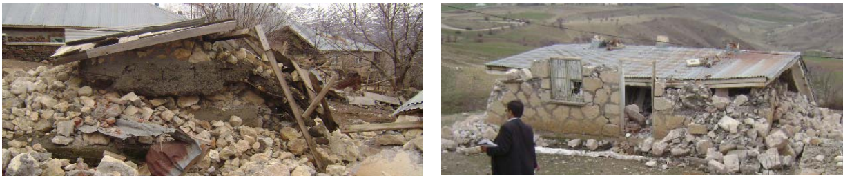
Figure 9 A heavy saddle shape roof
