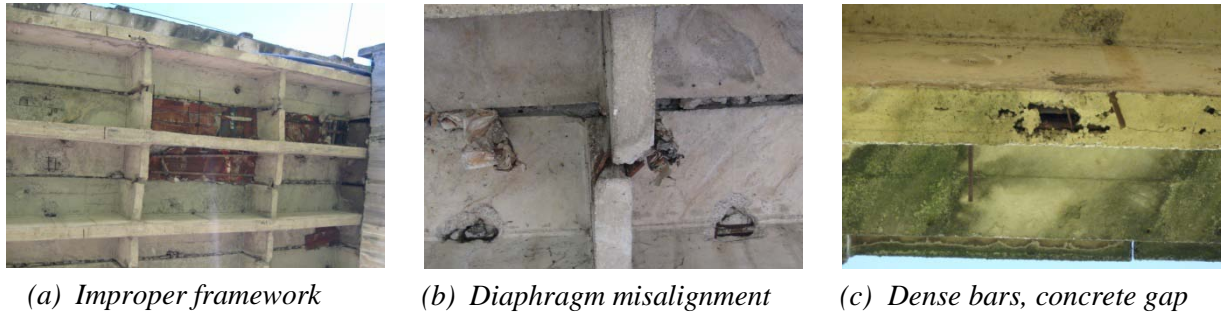
Figure 3 Deck defects
