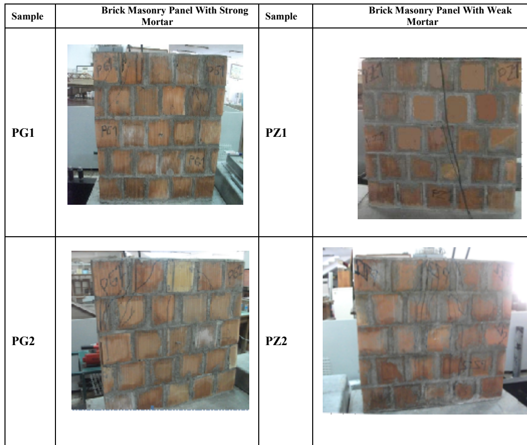
Figure 7. Apperance cracking of brick masonry panel with strong and weak mortars after loading
