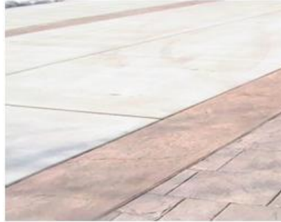
Figure 6: Concrete pavements with pattern
