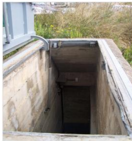
Figure 5: Utility Tunnel entrance from Barcelona – Spain (Canto-Perello et al., 2009)
