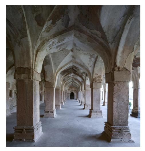
Figure 3: Lal Mahal. Western pavilion; main pillared hall based on the paratactic iteration of organically vaulted modules. (Photo by Fabrizia Dragone. February 2014)
