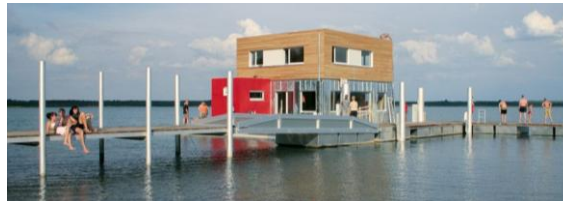
Figure 3: IBA Fürst-Pückler-Land, Germany 2000-10. Project 27: Floating Homes On Gräbendorfer See
