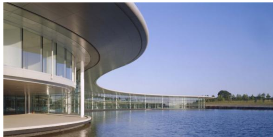
Figure 6: Foster + partners, McLaren Technology Centre, Woking, UK, 1998-2004
