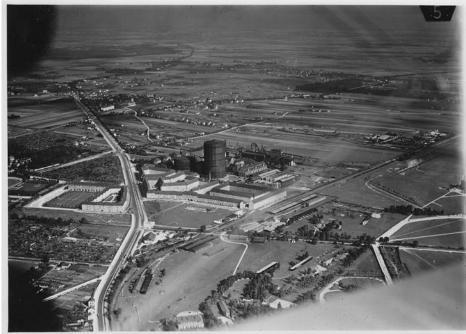
Figure 4: Aerial view gasworks Moosach/Borstei after 1931, schlot-Archive
