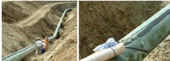
Figure 4: The temperature sensor cables on the gas pipeline SMARTape (Glisic and Inaudi, 2007; Nikles et al., 2004)
