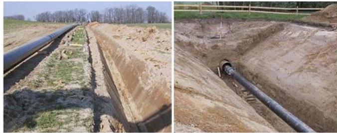
Figure 3: Fiber optic cables are laid below 10 cm of pipeline (Inaudi and Glisic, 2008)
